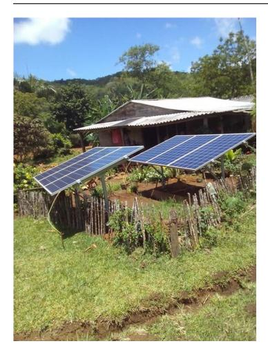
As part of the International Collaboration project with the Spanish Agency, it is intended to benefit 93 families in areas not served by the National Electric System in the municipality of Yateras, for them 52 isolated photovoltaic systems of 1.5 kilowatts (kW) were installed in Las Municiones, El Mosquito and La Demajagua communities.
